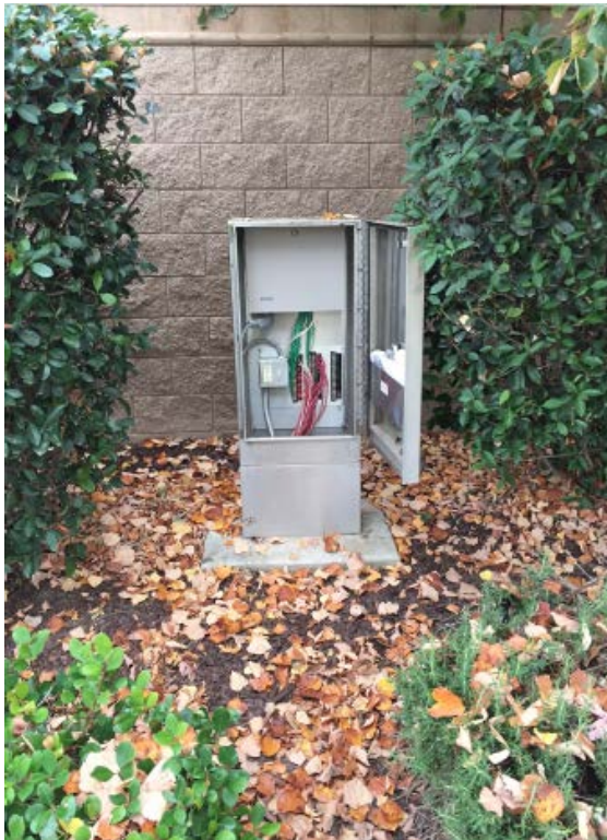
Stabler Lane at Rich Drive
